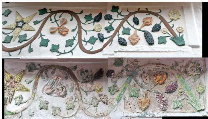
Work in progress on the pargeting
